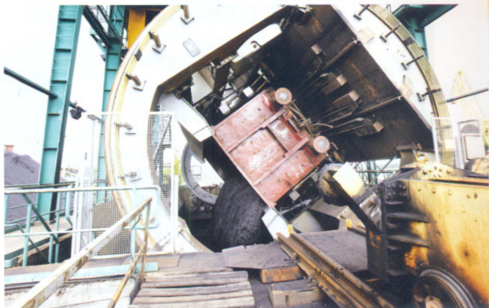
Wagon tipplers require a considerable amount of space.
