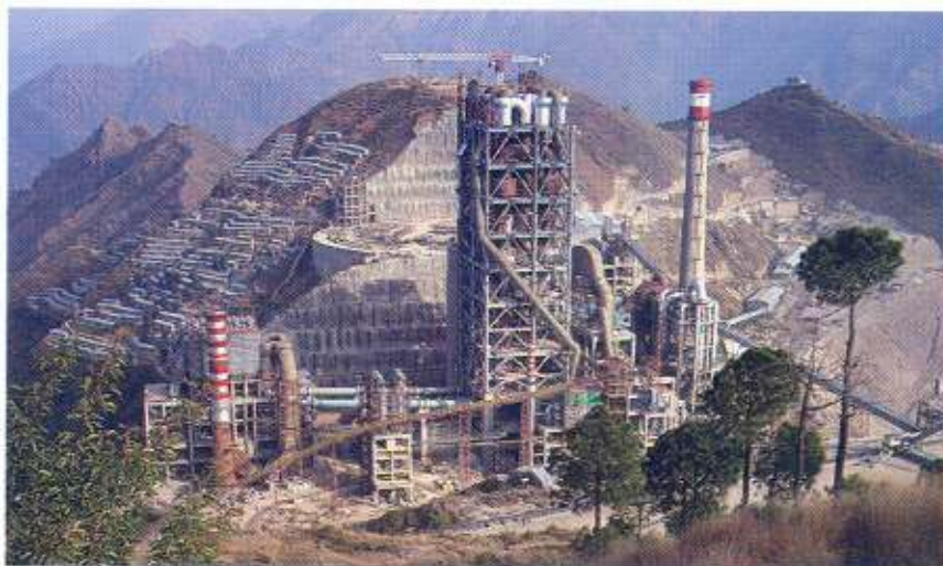
Jay pee Baga 10000 TPD Cement Plant
