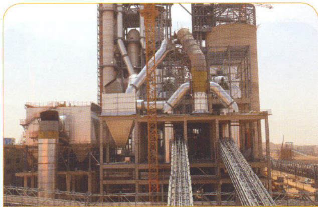
Process duct arrangement in raw mill area.
