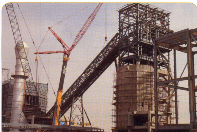
Deep pan conveyor for clinker transport.
