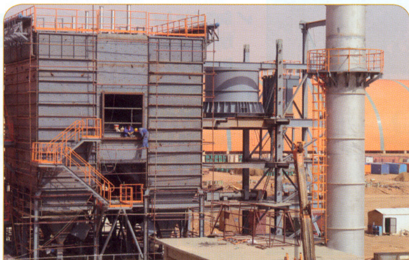
Bypass baghouse and structure.
